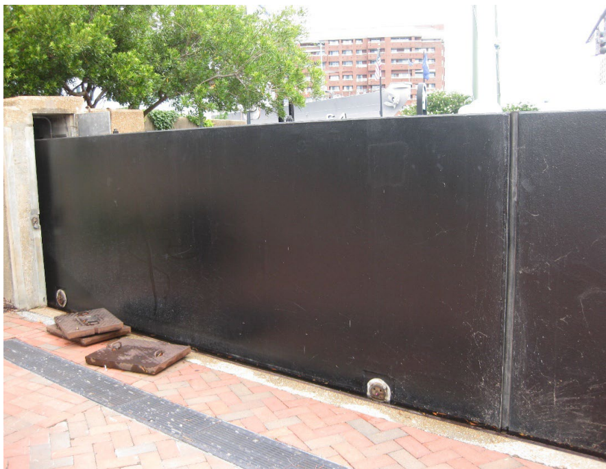
Figure 5.6.1.2.2: Slide Gate Example (Photo courtesy of USACE Norfolk District)
