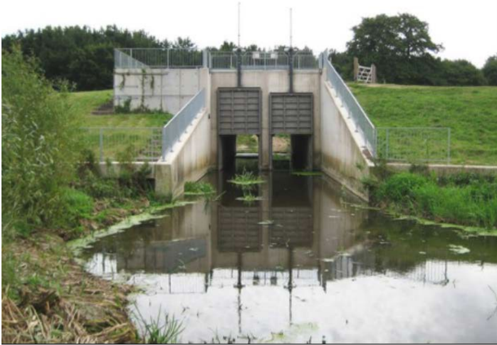
Figure 5.6.3.2: An Example of a Pair of Sluice Gates (Photo courtesy of USACE Norfolk District)
