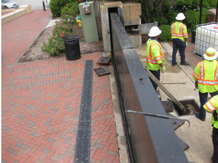
Figure 5.6.1.2.1: Slide Gate Example (Photo courtesy of USACE Norfolk District)
